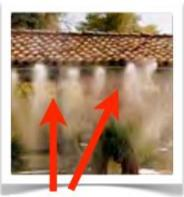
Effective cooling requires a **BALANCED nozzle placement** to eliminate **HOT Spots**. Each nozzle location has its' own area to cool, and improper placement **NEGATES** the available cooling effect.
